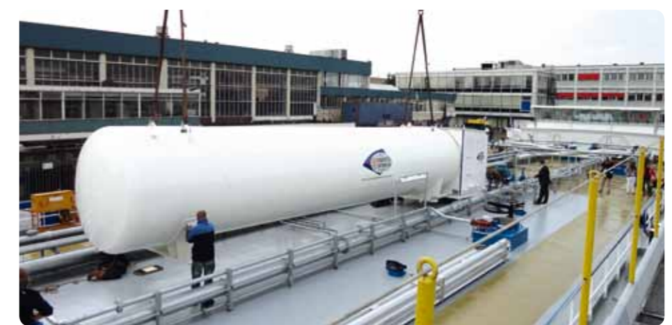
The LNG storage tank is lowered on to the Argonon chemical tanker (see LNG storage tank story by Lloyd's Register's risk expert Vince Jenkins)
