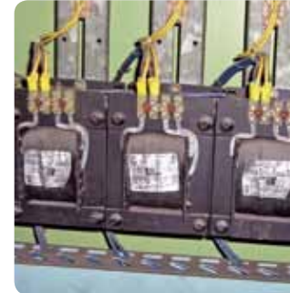
Old lighting ballasts on a ship may be contaminated with polychlorinated biphenyls (PCBs), which are persistent environmental pollutants.
